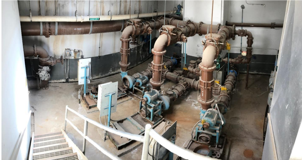
Figure 3-5: RAS/WAS Pump Station
