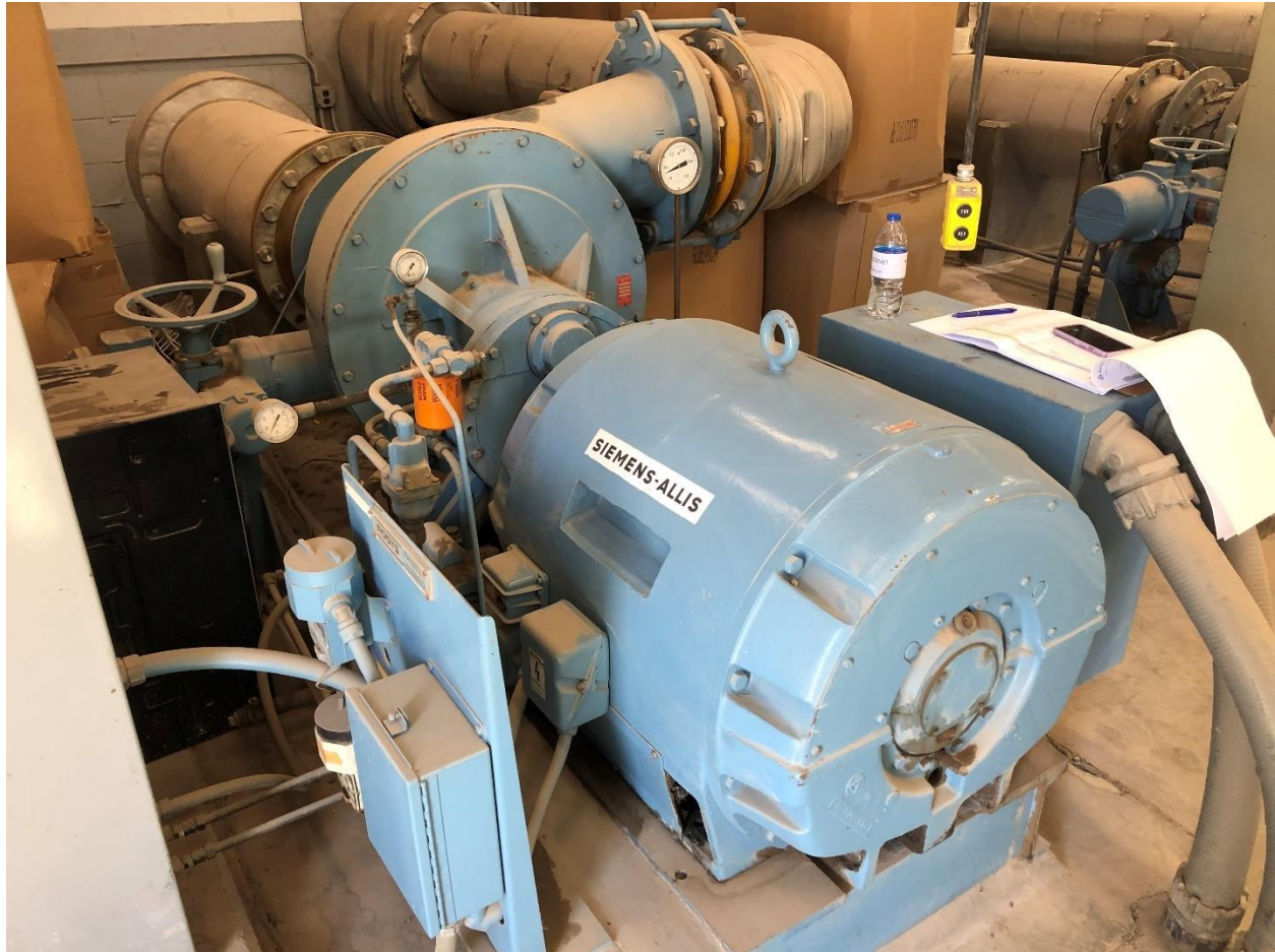
Figure 3-3: Aeration Blower Pump Motor
