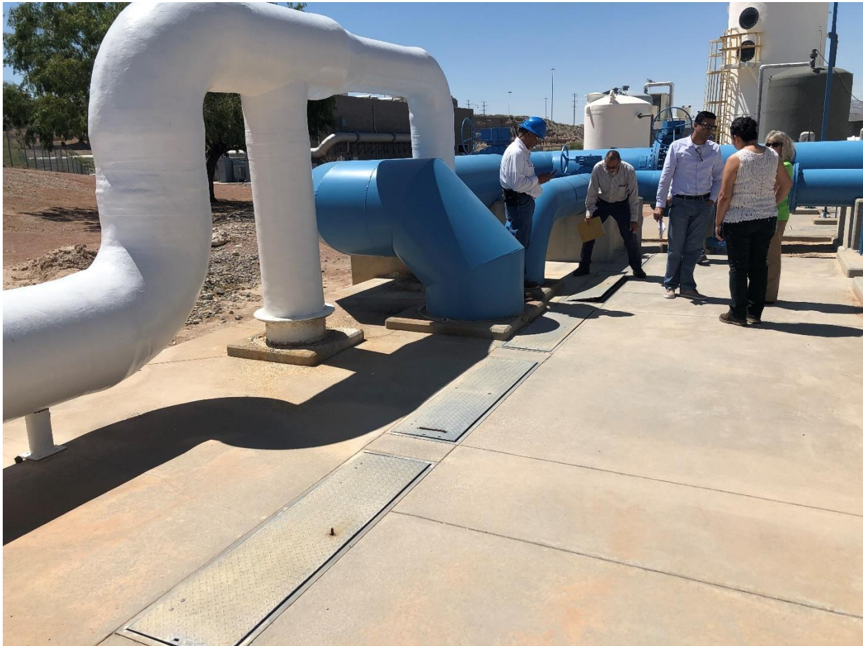
Figure 3-1: Aeration Splitter
