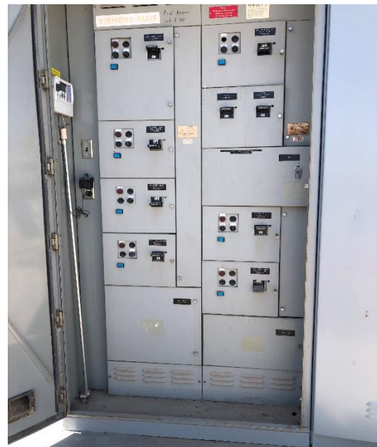
Figure 4-18: Existing Motor Control Center
