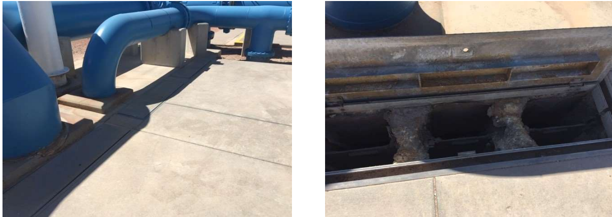
Figure A-2: Splitter Boxes Concrete Deterioration
