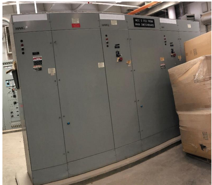
Figure 4-16: Existing Motor Control Center CB-MCC-5
