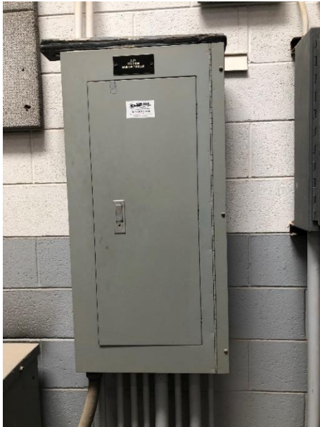
Figure 4-11: Existing Panelboard ELP1
