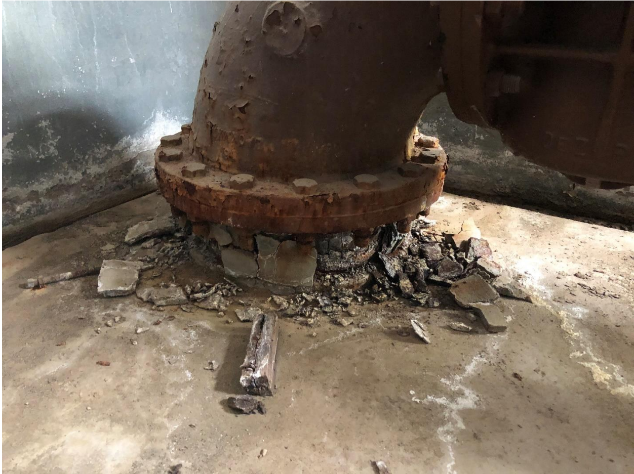
Figure 4-6: Concrete Deterioration around RAS Pump Piping
