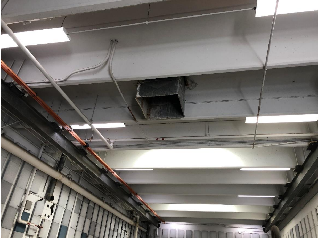
Figure 4-3: Intake Box Filter in Blower Building
