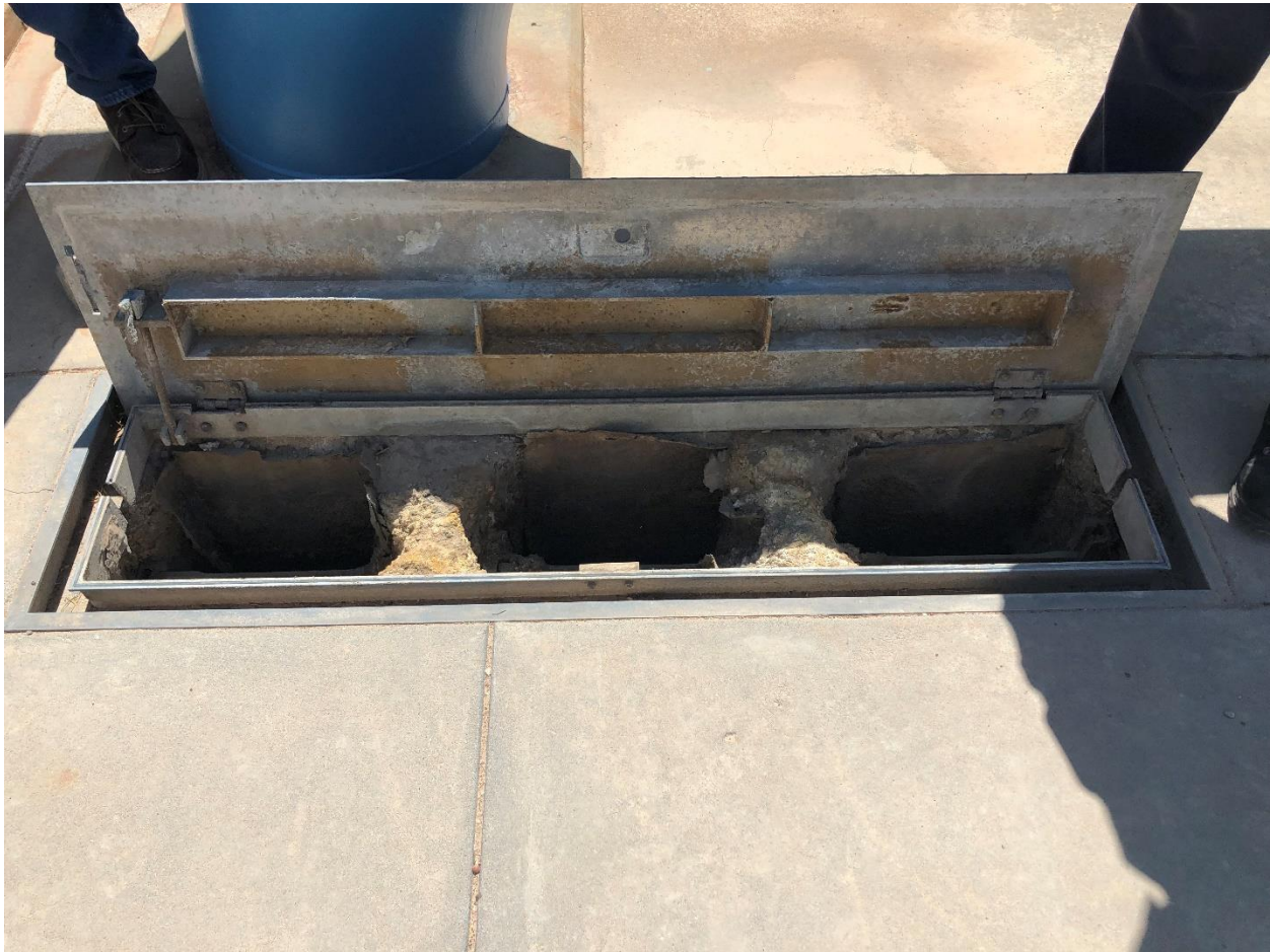
Figure 4-1: Splitter Box Concrete Deterioration
