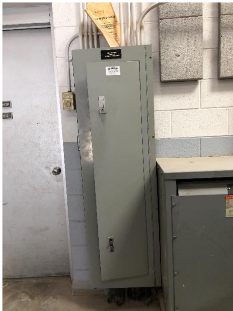
Figure 4-17: Existing Panelboard LP2
