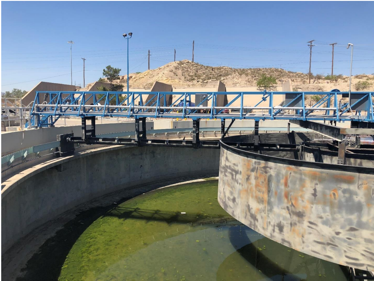
Figure 4-4: Non-operational Secondary Clarifier Arm
