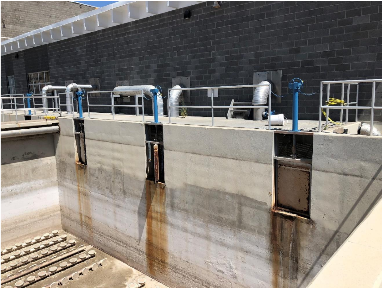
Figure 4-2: Aeration Basin Butterfly Gates
